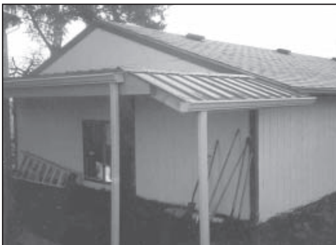
New porch to divert water away from the building
